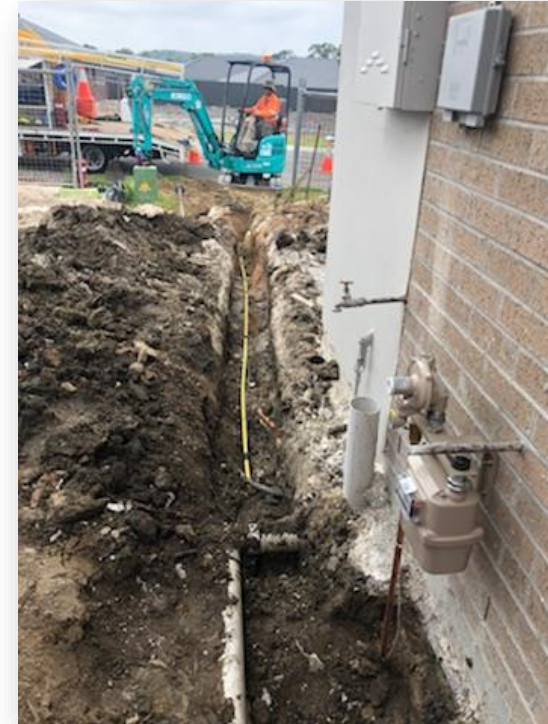
Example of a connection to a residence (a basic connection)
