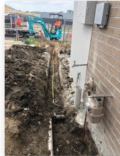
Example of a connection to a residence (a basic connection)
